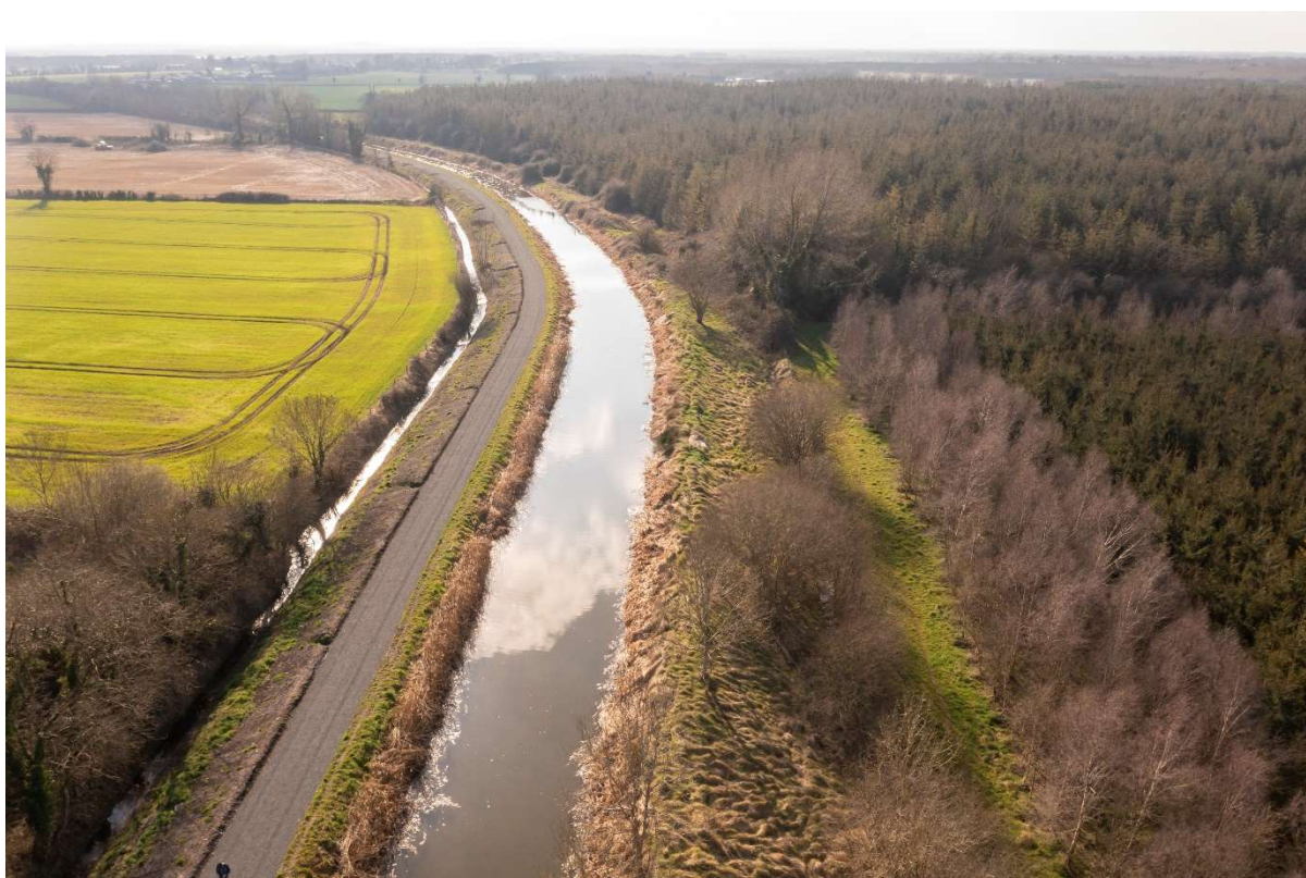
Fig 1 – Aerial photo of works south of Wilsons Bridge
