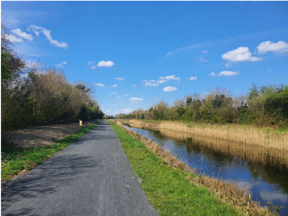
Fig 2 – Vicarstown – Courtwood following completion
